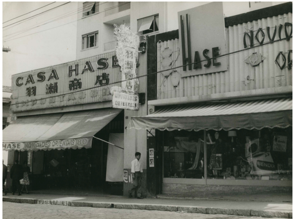
Fig. 11 — Dilson Martins, untitled, Detail for the Casa Hase building façade (with different types of signs for the Japanese products store), c. 1970. Correio da Manhã Collection, Arquivo Nacional.
